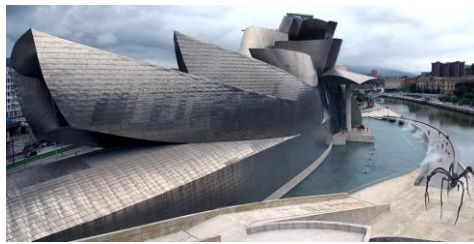
Fig. 1: Guggenheim Museum, Bilbao-Spain, 1993-1997 [20].
