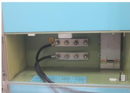
Fig. 3: Impulse Generator for High Current
