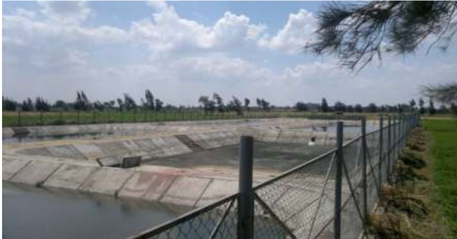
Fig 1. Quleaa SPO Plant at Kafr ElShiekh , Egypt with 500m 3 /d Capacity.
