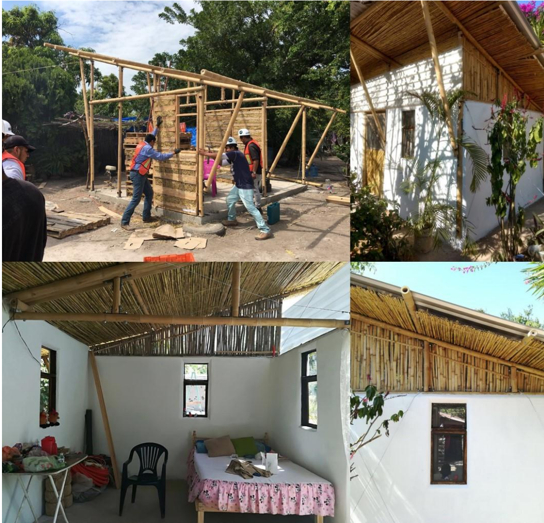
Fig. 2: Clockwise from top left: Scholars and brigades building a bamboo structure and pallets envelop; top right: House 1 with finished plaster and painting; bottom right: A detail of a weaving layer for roof insulation of local reeds and window made of re-usable wood from pallets; bottom left: Detail of the interior of house
